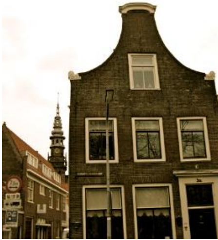
Figuur 23, Houten afdekking, pand Haarlem
